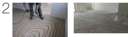
SISTEMI AD ACQUA CALDA: - SISTEMI A SECCO
